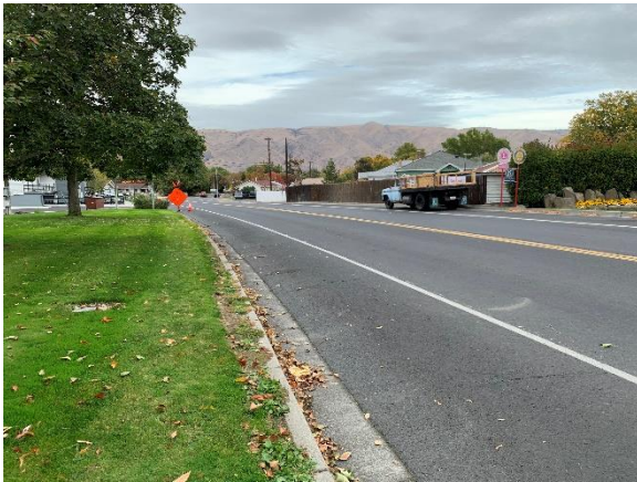
5 th Street Facing North
